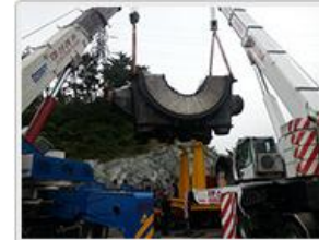
Seating the Exist LP Lower Casing
