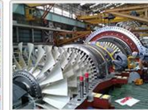
Blade Ring Assembly & Bolt Tightening
